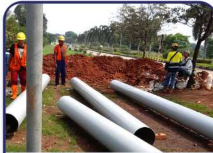
Proyek Pipa P8
