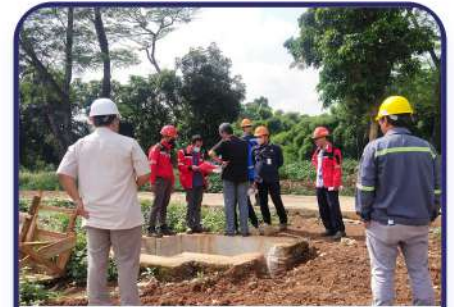
Proyek Pipa P8
