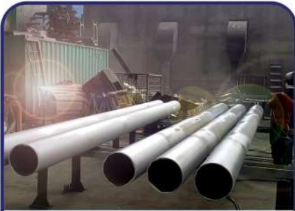
Proyek Pipa P8
